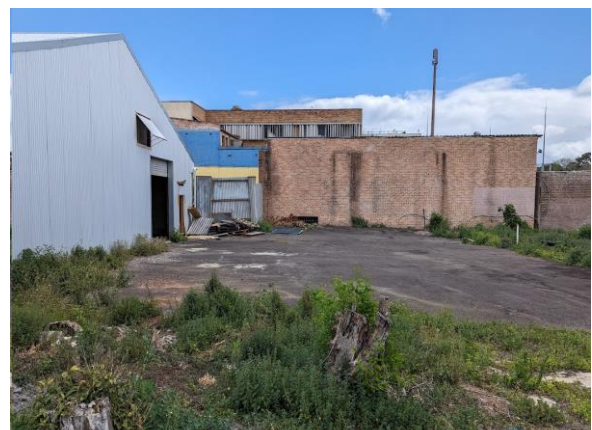
Overland flowpath through buildings and fences near Parramatta Road, viewed from Coles Street, Burwood Precinct
